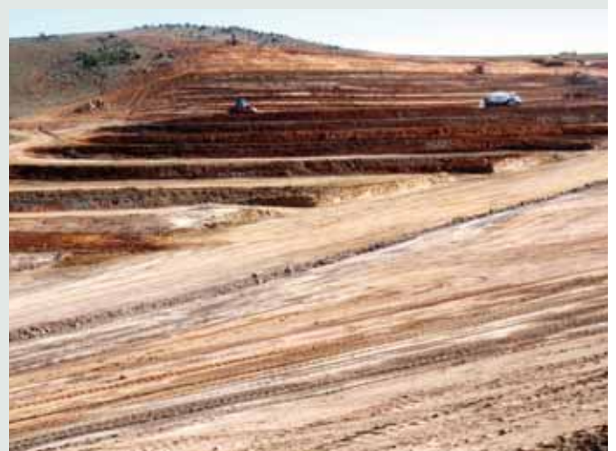
Central Valley Earthworks
